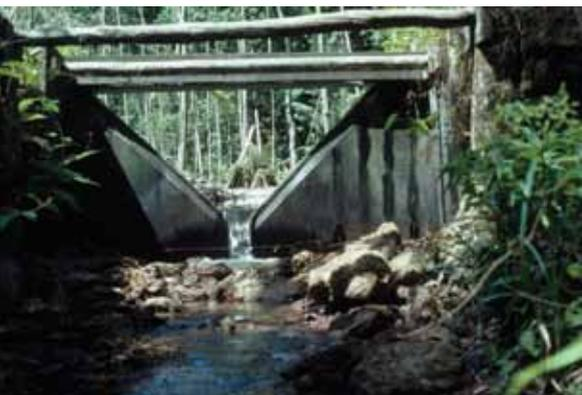
Photo 6.2. Weir to measure water flow, Kabo, 1982.
